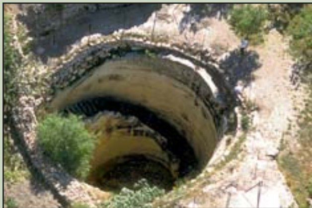
The Pool of Gibeon was a massive 37-foot diameter shaft cut into solid rock to reach the water table 82 feet below.
